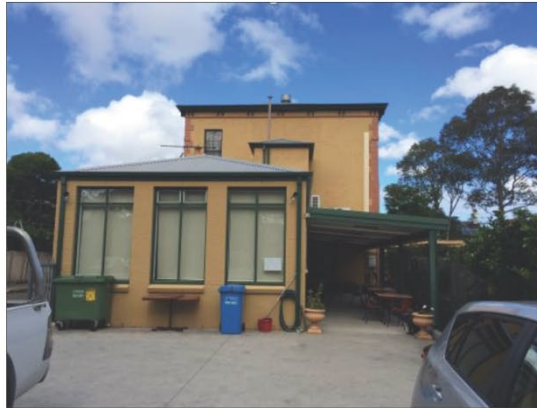
Figure 9: Rear (western) elevation.
