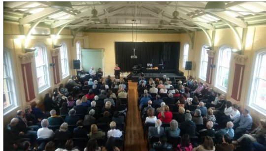
Figure 11: Hall looking north west, showing the roof structure. Greek Atlas League.
